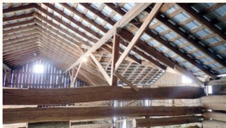
The logs used to construct the barns were typically sourced locally from the property. The wood was then hand hewn, meaning they have been flattened and squared using hand held tools. Because the process is performed by hand, the finished edges of the wood is often rough and choppy. This roughness provides a “rustic” appearance that is cherished today.
