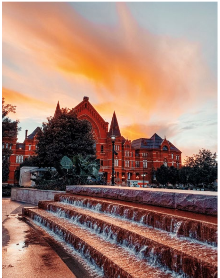
A view of the Cincinnati Music Hall from inside Over-the-Rhine's Washington Park.
